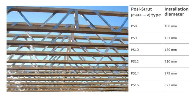
The open diagonal design gives plenty of room to run water, sewage, and ventilation through the beams, without cutting and drilling.
